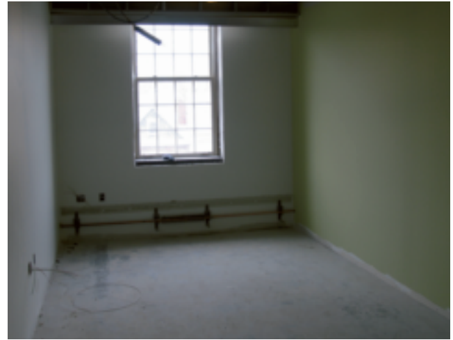
West-side office in top floor of 1985 structure.
