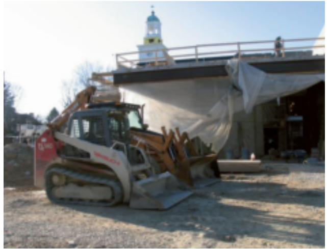
The new classroom addition in progress viewed from the north side.
