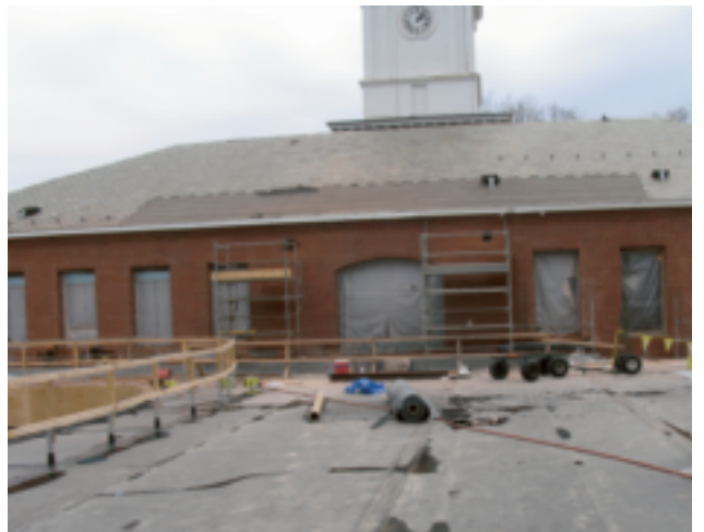
Soon-to-be green roof connecting to west side of Trickett Hall.
