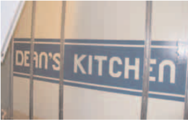
Wall uncovered during work on the interior of Trickett Hall
