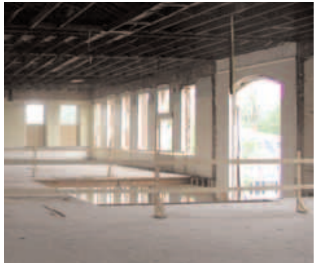
Second floor of Trickett Hall
