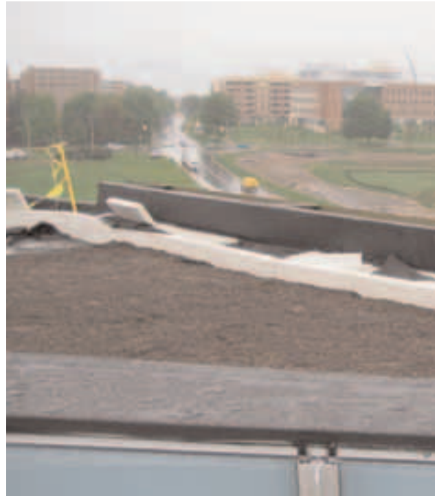
View of green roof atop Lewis Katz Building
