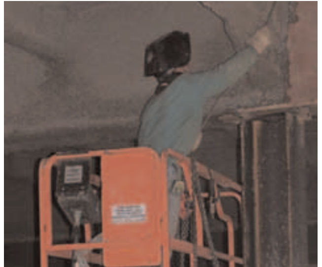
Worker scraping fireproofing material from 1985 addition
